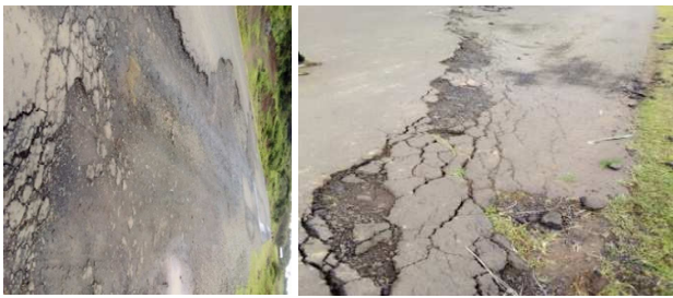
Figure 11. Distresses on selected segment (photo: by Mengistu Bayu, 28 th May, 2021).
