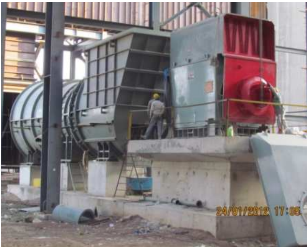
Figure 1. Typical ID Fan resting on Foundation.
