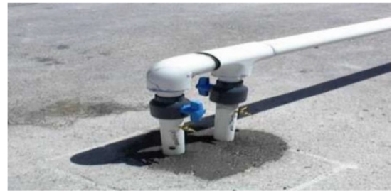
Figure 2. Typical pipes transporting vapor from the underground SVE well to treatment [34].
